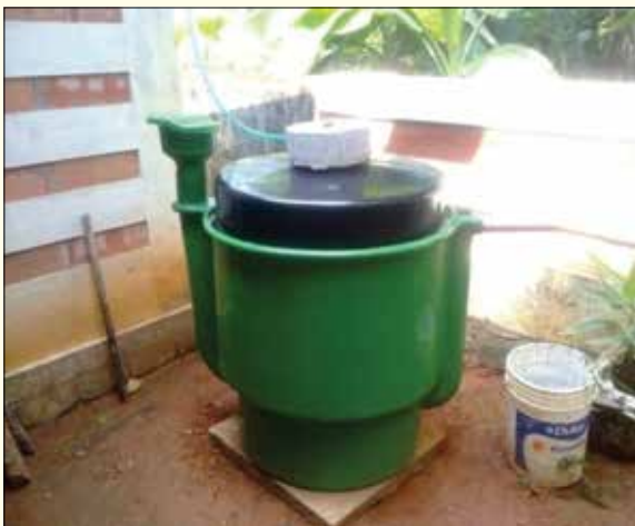
Figure 3.17 Portable Household Biogas Plant
